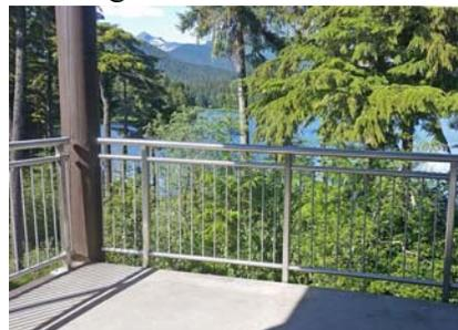
These guardrails meet current building codes, unlike our old ones. They are made of Stainless Steel and will never have to be painted. The old wood rails required re-painting every 10-15 years and it took a ton of labor to prepare all of
