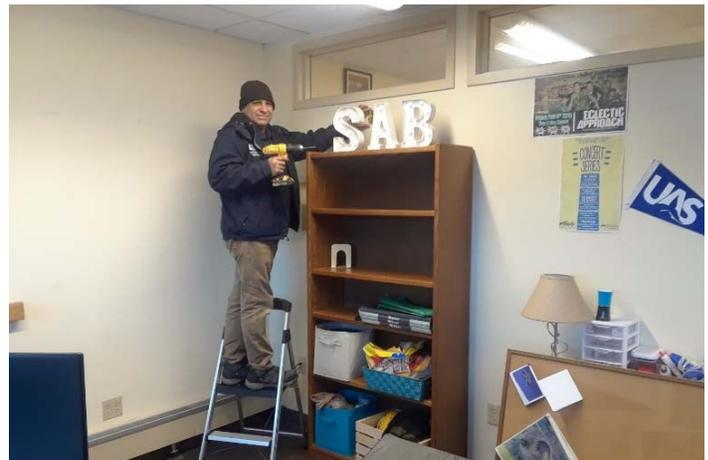
*UAS Facilities Maintenance Carpenter Jose Islas is pleased to be securing a tall wobbly shelving unit to the wall. Note that he is locating the stud in the wall prior to installing the fastener.*
