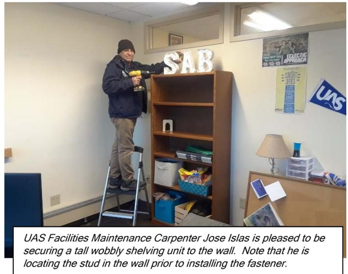
*UAS Facilities Maintenance Carpenter Jose Islas is pleased to be securing a tall wobbly shelving unit to the wall. Note that he is locating the stud in the wall prior to installing the fastener.*
